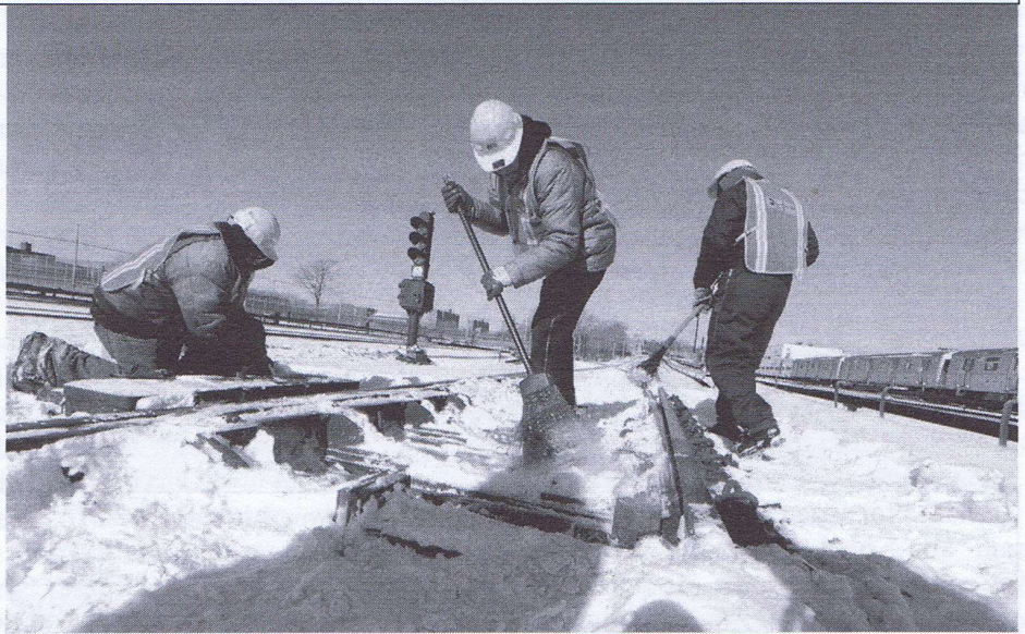
Cleaning a switch the old way—by hand.
