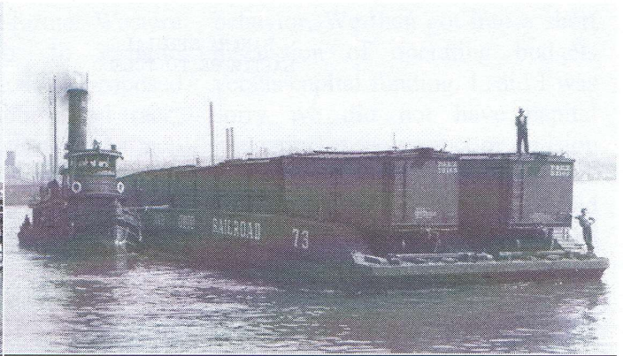
The B&O tug Baltimore , a steam-power tug, unlike the diesel-power George M. Shriver in the picture on the left, is shown with a carfloat of Fruit Growers Express refrigerator cars on Carfloat #73. Each carfloat could carry five cars on each of the two tracks. Based on the clothing on the deckhands, it must be warm weather and probably in the 1930s.
