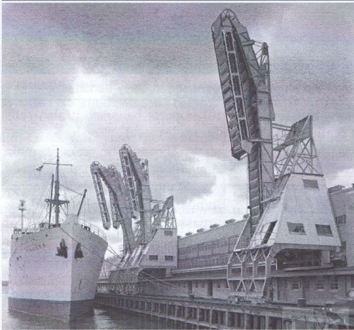
Photos of the machinery used to unload the ships and the “curveyors” used to carry the bananas to the railroad cars for loading.
