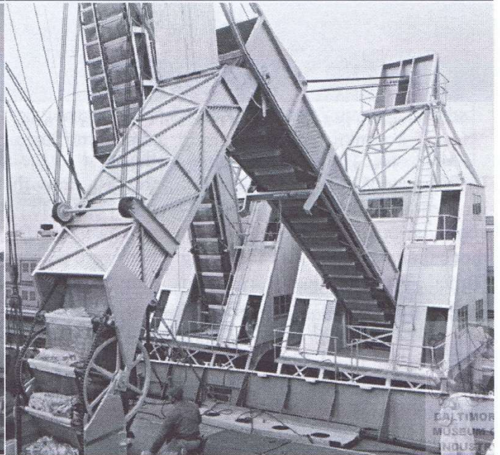
Photos of the machinery used to unload the ships and the “curveyors” used to carry the bananas to the railroad cars for loading.
